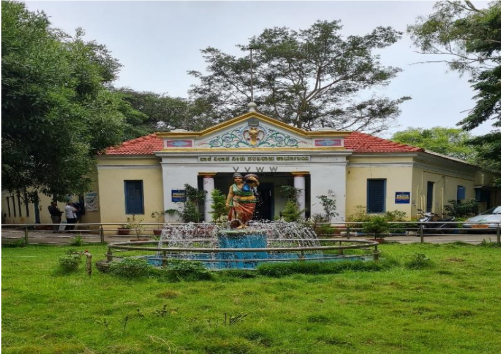
Vanivilas Water Works
