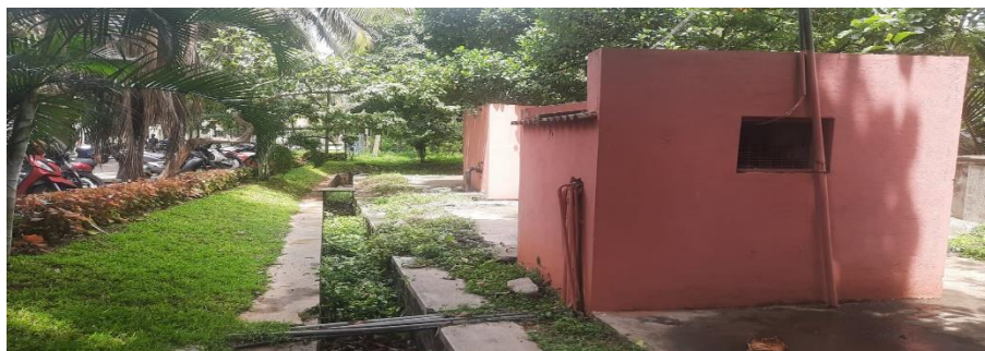
Waste water storage facility
