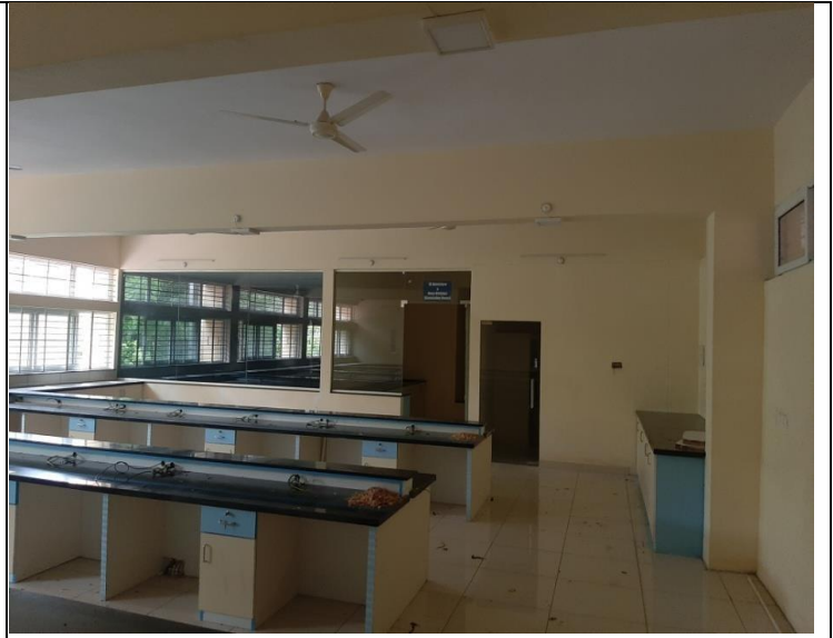
Renovation of Microbiology Laboratory
