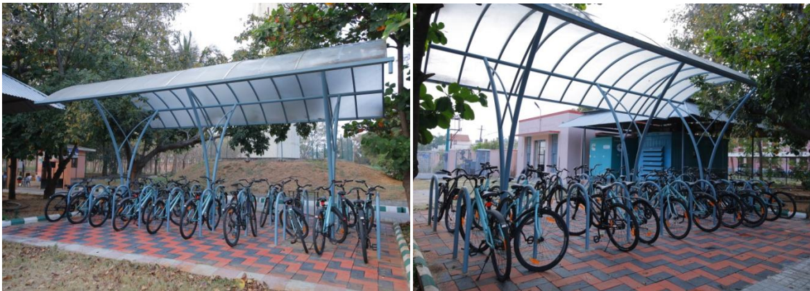
Bicycle stand constructed within the campus
